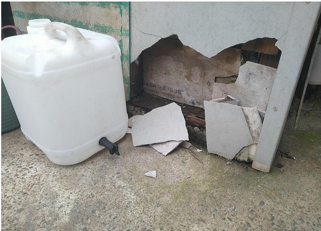
Photo 8: Potential asbestos containing materials at rear of property
